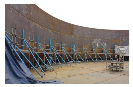
Jacking Equipment for erecting Storage Tanks has been in the market for over 10 years. Jacking system will allow construction time to be reduce by 40% and it will minimize cost, labor and risk of accidents.
